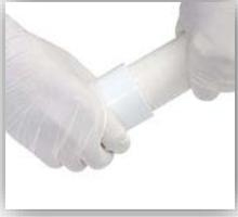
Check pipe and fitting for proper dry fit before cementing. For a good interference fit, the pipe should easily slip into the fitting 1/3 to 2/3 of the way. Too tight of a fit is not acceptable because the pipe may not be able to bottom into fitting during assembly.
