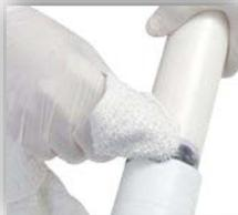
Using a rag, remove the excess cement from the pipe and fitting.
