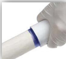
Hold the pipe and fitting together for at least 30 seconds to prevent movement or push-out. Check around top of joint for a ring or bead of cement. If there are gaps or voids in this bead, sufficient cement may not have been applied and the joint may be defective and leak.
