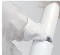
Using a rag, remove the excess cement from the pipe and fitting. This bead or excess cement is not needed and will not provide extra strength in the joint and will extend the set and cure time.
