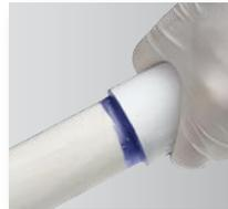
Hold the pipe and fitting together for at least 30 seconds to prevent movement or push-out.
