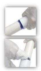
Hold the pipe and fitting together for at least 30 seconds to prevent movement or push-out. Check around top of joint for a ring or bead of cement. If there are gaps or voids in this bead, sufficient cement may not have been applied and the joint may be defective and leak.
